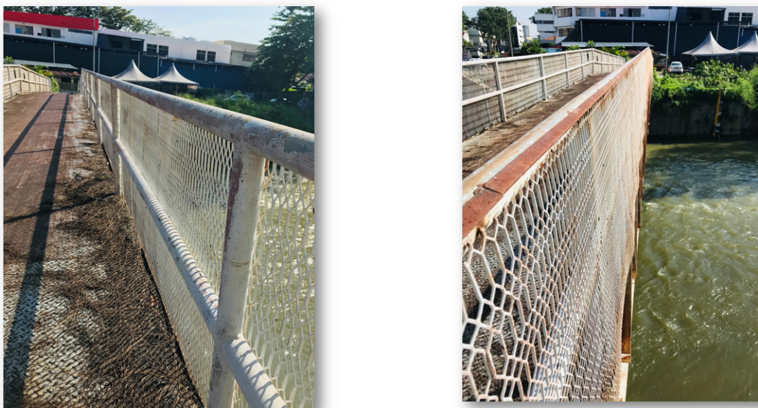
Figure 19: Steel Bridge Safety Railing
