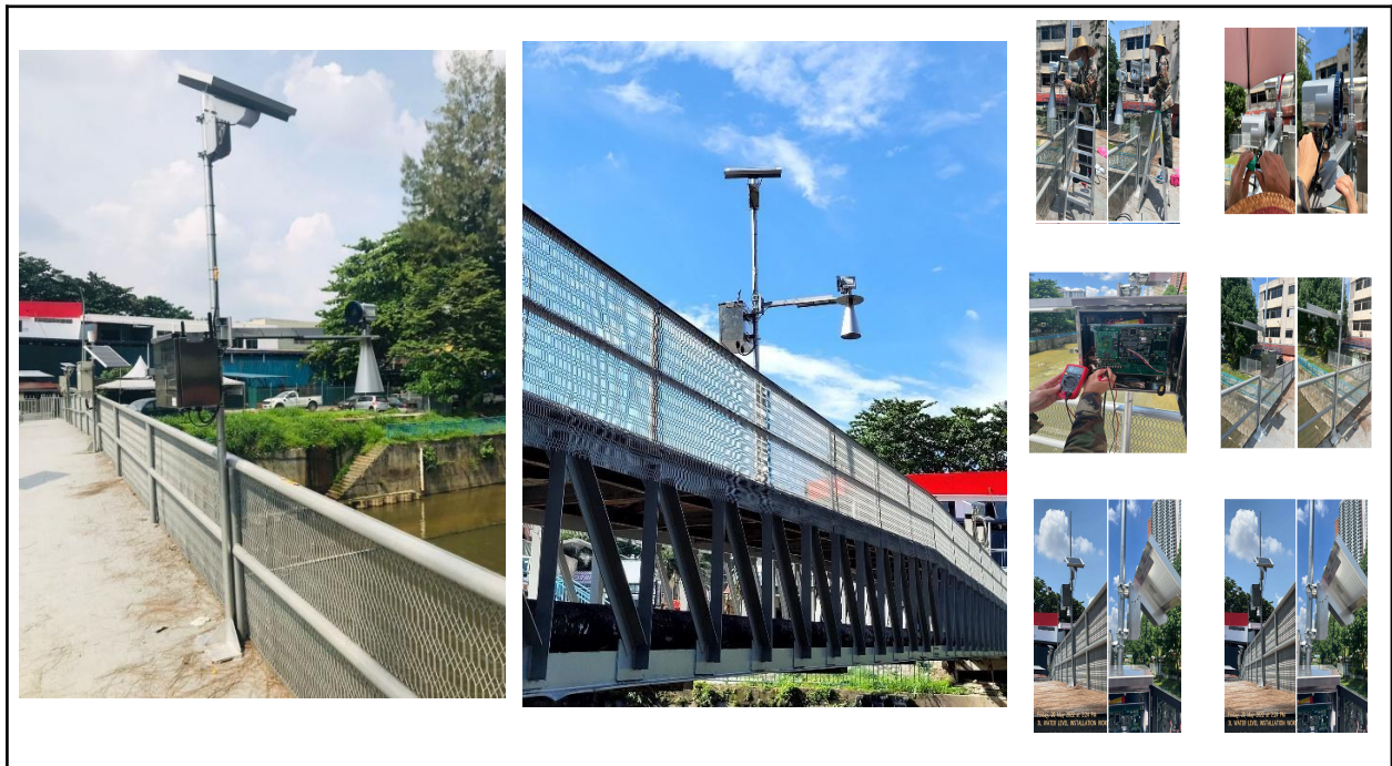
Figure 22: Picture of WLG Installation Progress of MEISEI ELECTRIC CO., Ltd.
