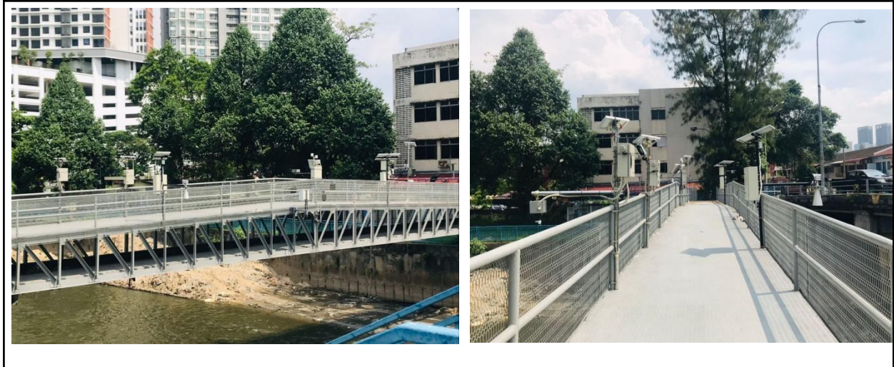
Figure 20: Picture of all WLG installed at site
