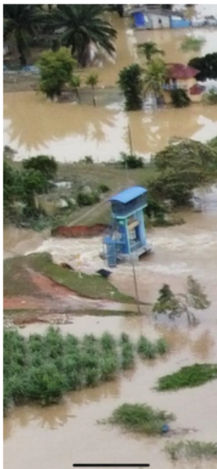
Tidal Gate Breach
