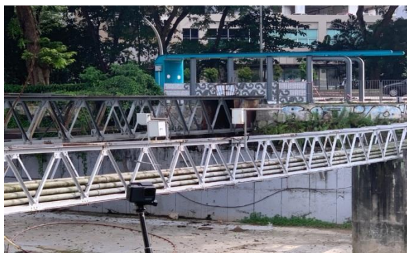
Figure 15-A: Sulaiman Bridge Station
